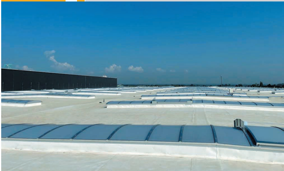
FOT. 2. Cool roofs MAN Poland
